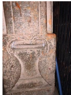
Photo 17: Right jamb of door-1
