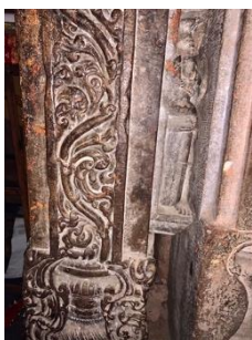
Photo 18: Left jamb of door no. 2
