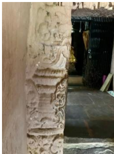
Photo 16: Left jamb of door-1
